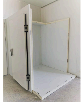
Room with floor panel during assembly
